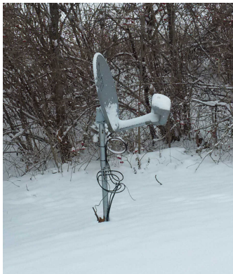
Figure 4.6: A snow covered dish antenna.
